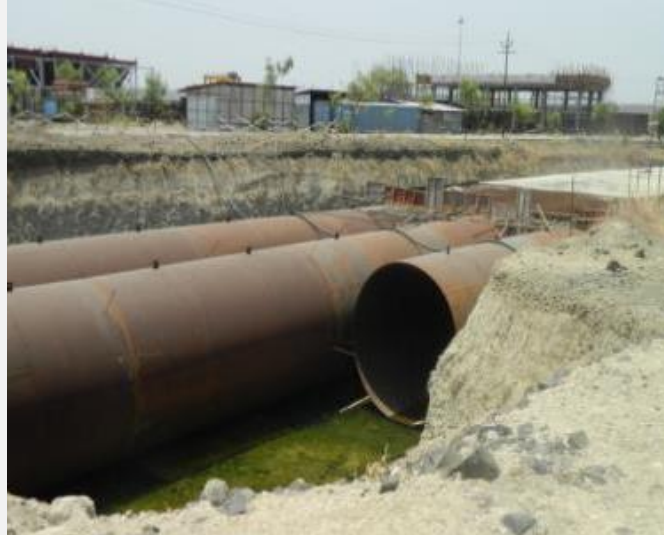
CW Piping with Encasing
